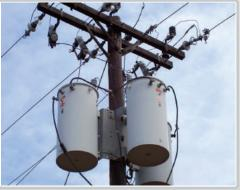
These crimped connections between these transformers appear to be loose. They should be checked. A failure here would shut down the entire plant.
